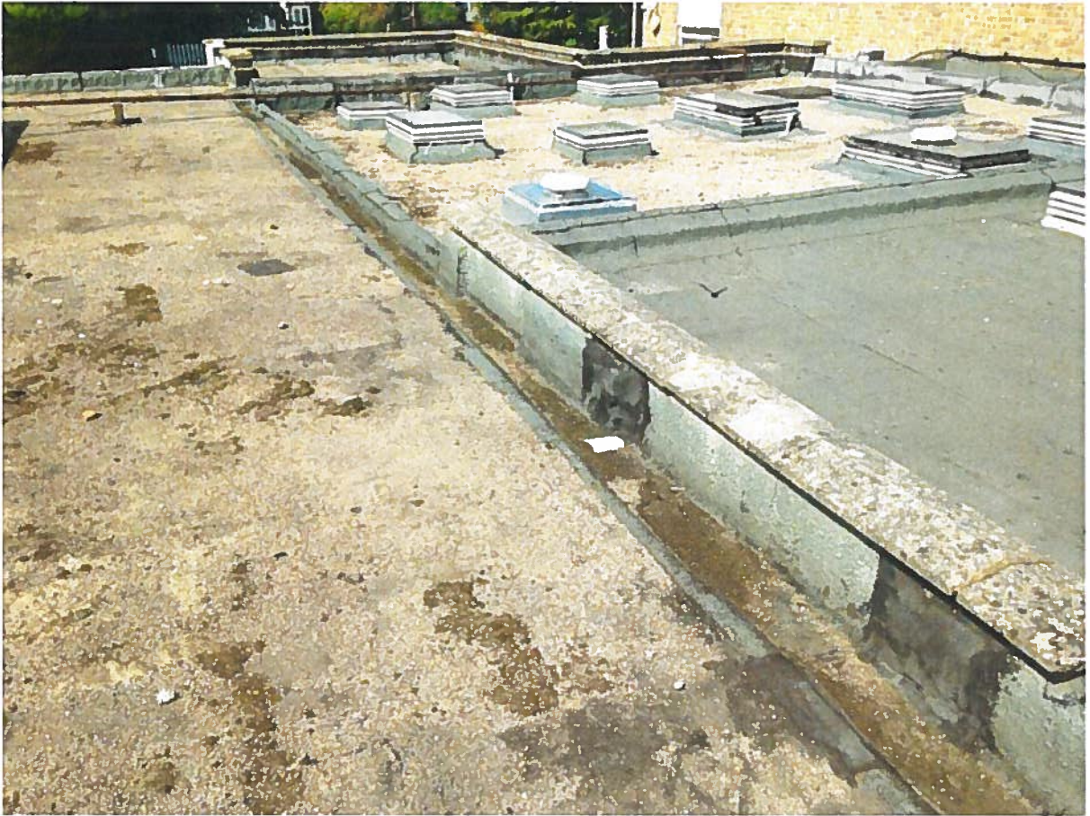
View from roof 5.jpg
